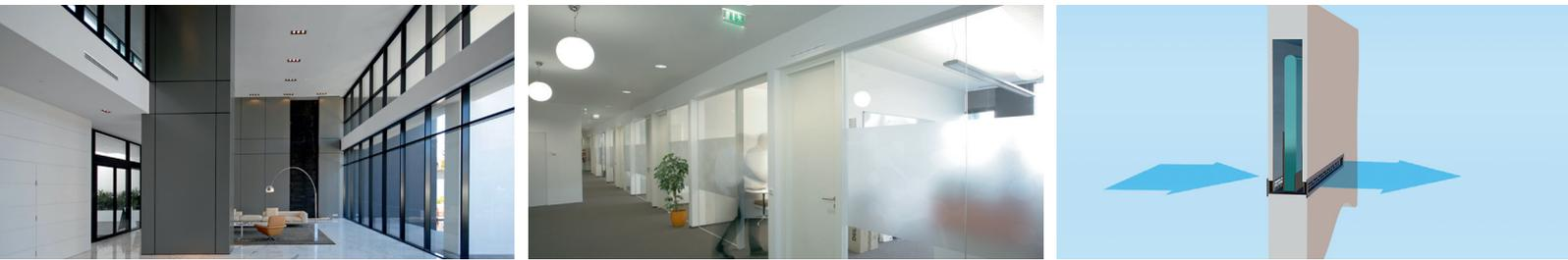
LDO-T air transfer devices provide significant cross-talk attenuation between adjacent rooms, whilst ensuring safe air transfer and limiting pressure differentials between rooms.
