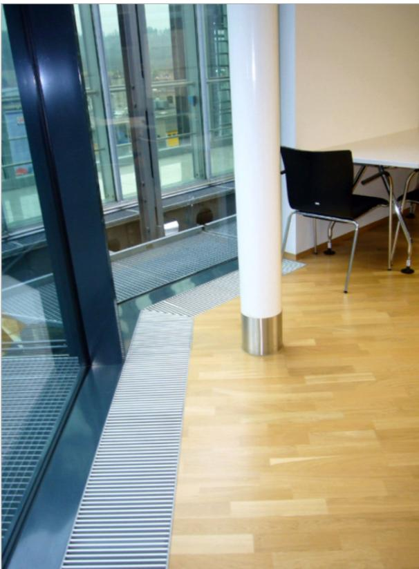
*Installation example, with LTG aluminum roller grille*
