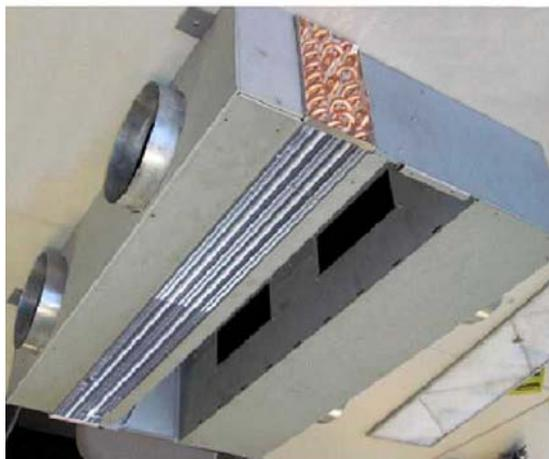
3. Removal of lower plate / vacuum-cleaning of heat exchanger on the pressure side
